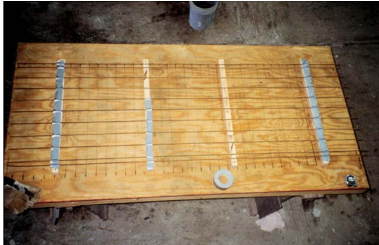
Figure 4.14 Process Used to Build the Curtains of Longitudinal Reinforcement
