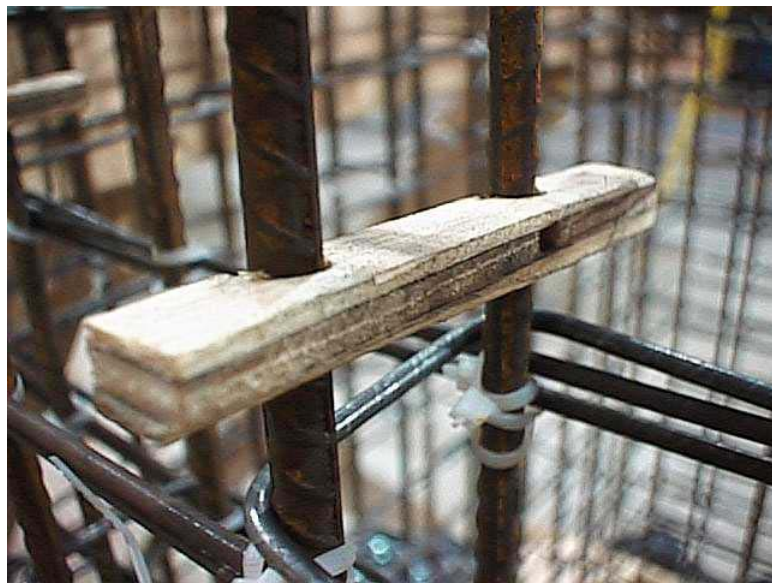
Figure 4.19 Spacer Used to Separate Exterior and Interior Forms
