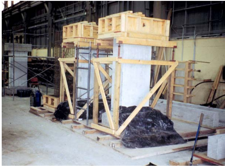
Figure 4.20 Top End Block Forms
