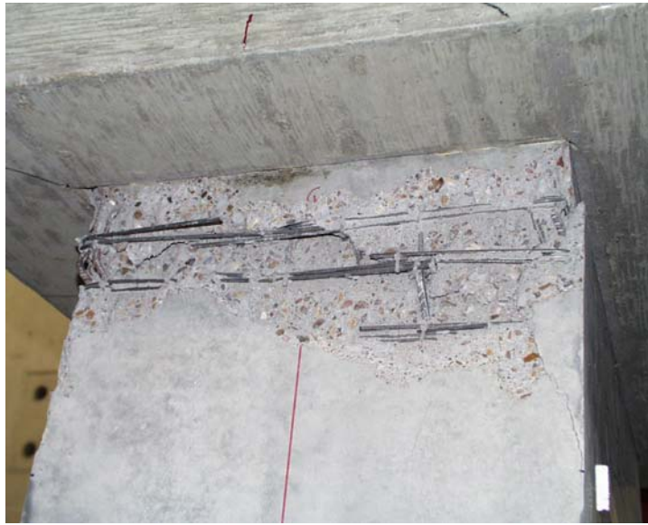
Figure 5.60 Specimen P14: Photo of North Wall at End of Test
