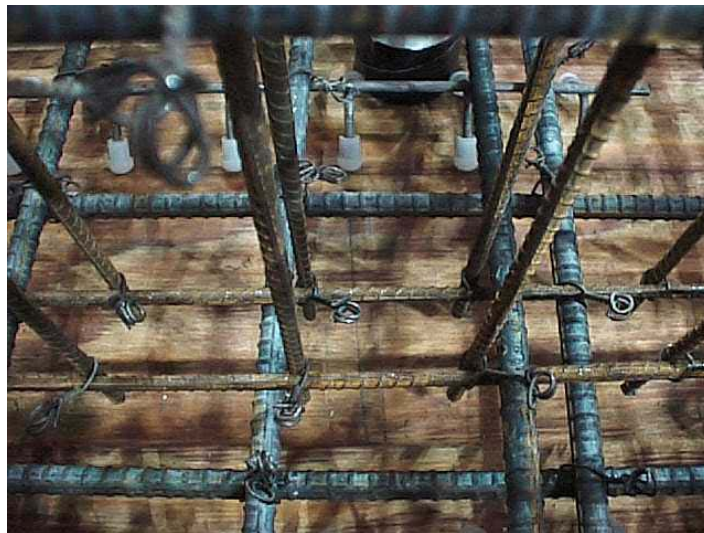
Figure 4.15 Alignment of the Longitudinal Reinforcement
