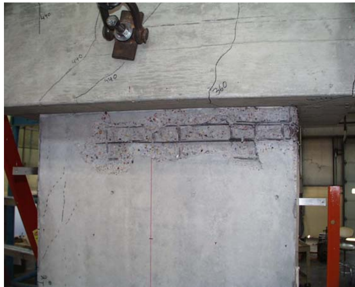
Figure 5.59 Specimen P14: Photo of East Wall at End of Test
