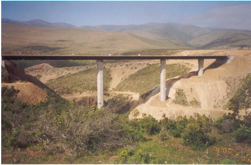
Figure 1.1 Bridge Puente Amolanas, With Three Hollow, Octagonal Concrete Piers
