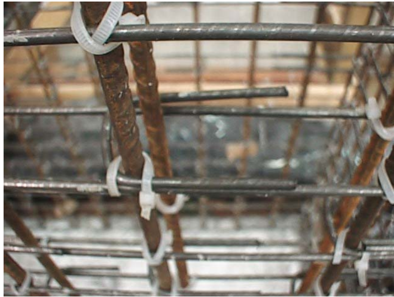
Figure 4.9 Typical Cross-Tie
