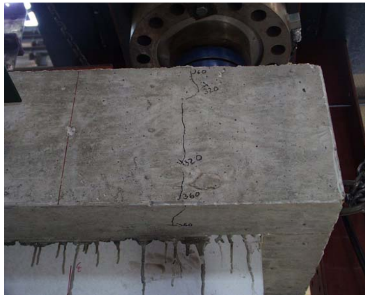
Figure 5.22 Specimen P8: Vertical Crack at East Side of the Top End Block
