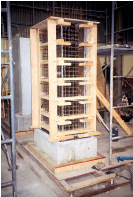
Figure 4.18 Exterior Forms on a Pier
