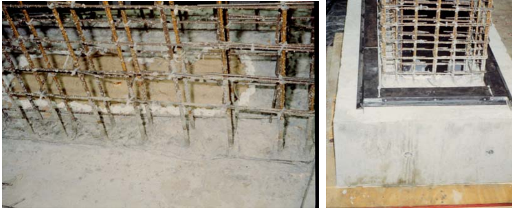
Figure 4.17 Sand and Neoprene Pads Used as Support for the Pier's Formwork
