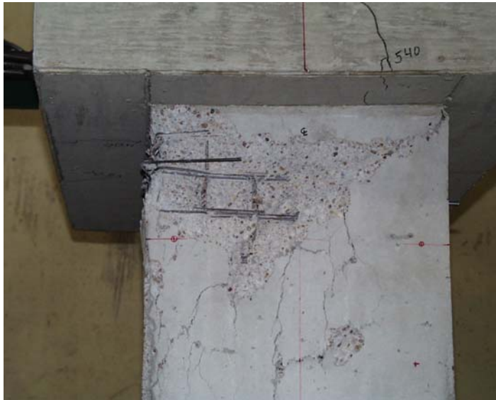
Figure 5.5 Specimen P6: Photo of North Wall at End of Test
