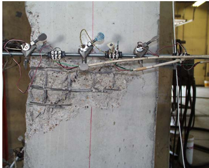
Figure 5.20 Specimen P8: Photo of North Wall at End of Test
