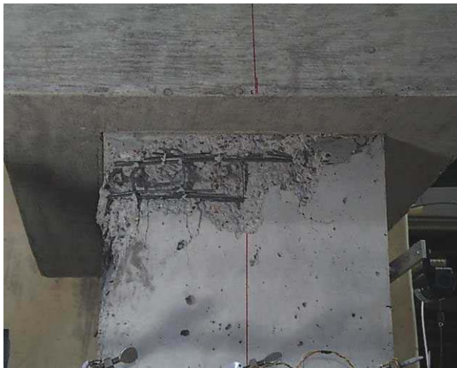
Figure 5.32 Specimen P10: Photo of North Wall at End of Test
