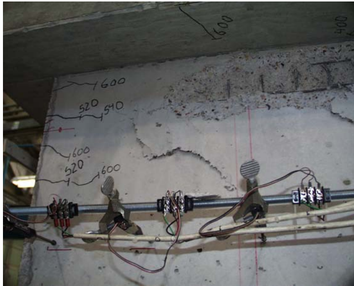
Figure 5.9 Specimen P6: Cracks and Crushed Concrete at South End of East Wall
