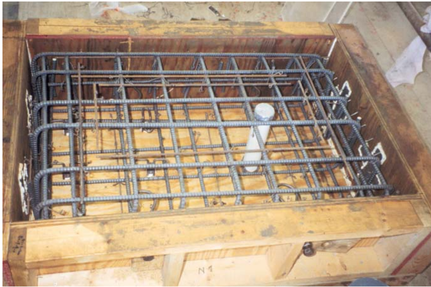
Figure 4.13 Reinforcement Cage of Bottom End Block
