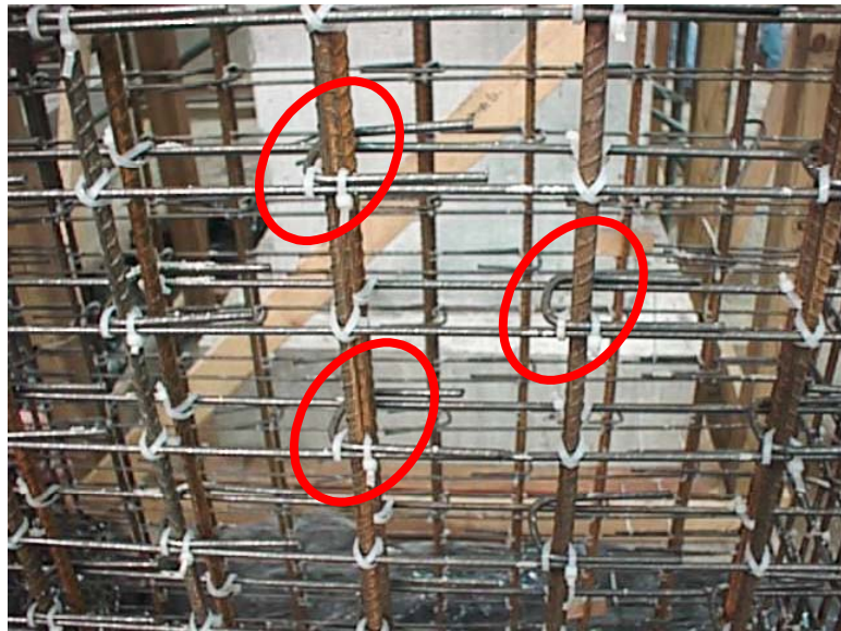
Figure 4.10 Checkerboard Pattern Distribution of Cross-Ties
